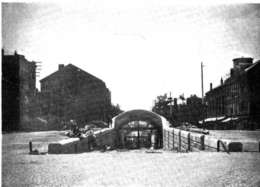
APPROACH TO THE BOSTON TUNNEL, MAVERICK SQUARE.
