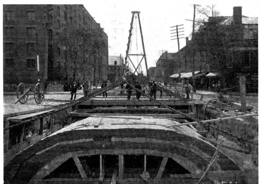
THE MONOLITHIC, CONCRETE, ROOF OF THE TUNNEL.
