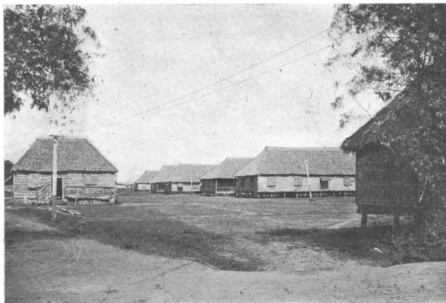
Bamboo and Thatch Barracks for 1,200 Men Built by Chinese Contractor in 23 Days.
