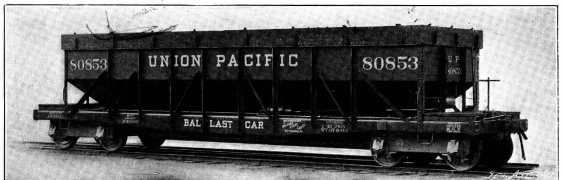
Ballast Car—Capacity, 100,000 Pounds; Weight, 37,600 Pounds.
