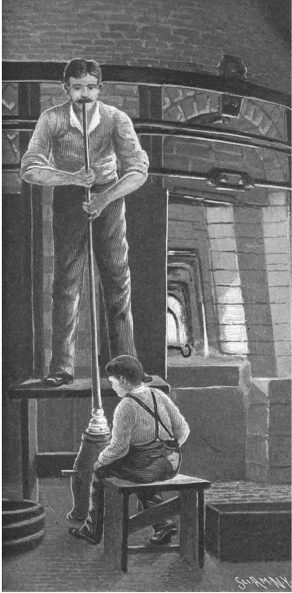
Forming the Chimney in the Mold.
