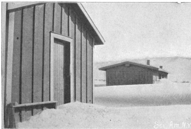
SAND DRIFTS AT RIMLON, CAL.
