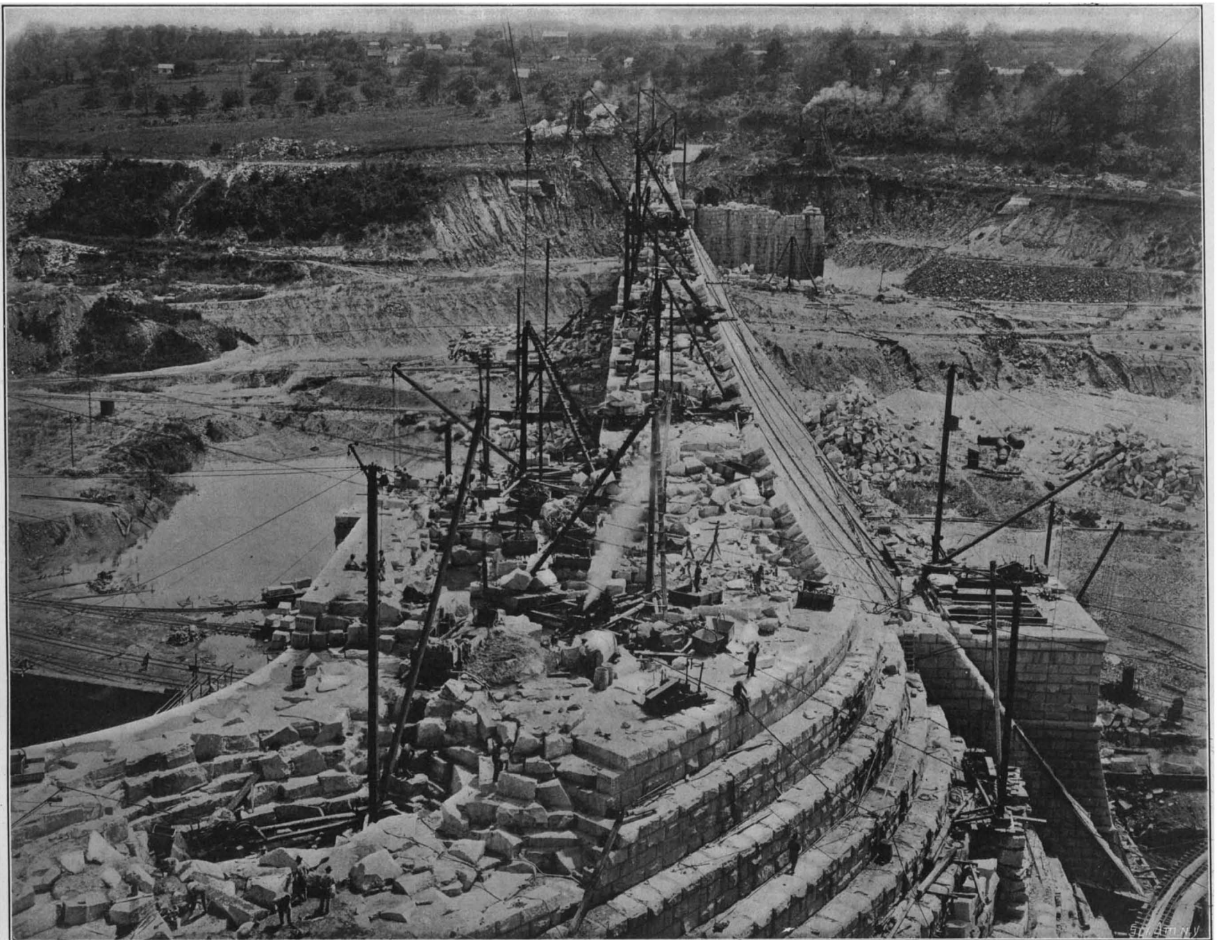
The Downstream Face of the Dam, Showing Commencement of Spillway and Headgate.
