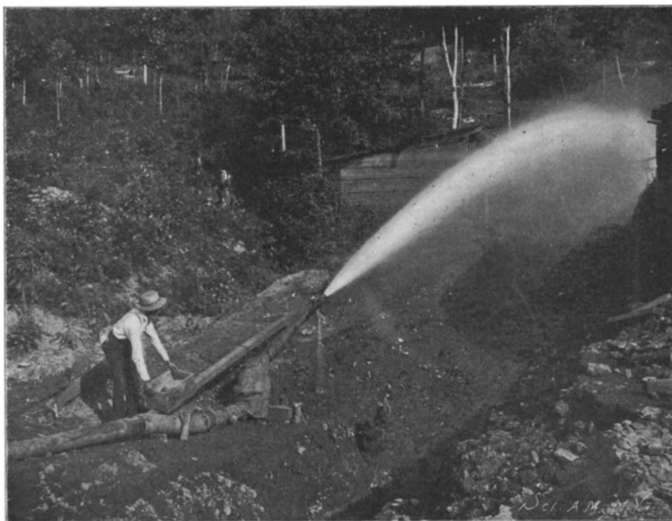
AN HYDRAULIC MONITOR AT WORK.
