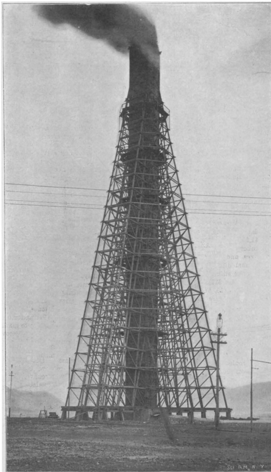
Interior dimensions, 10 feet by 10 feet; height, 180 feet.
