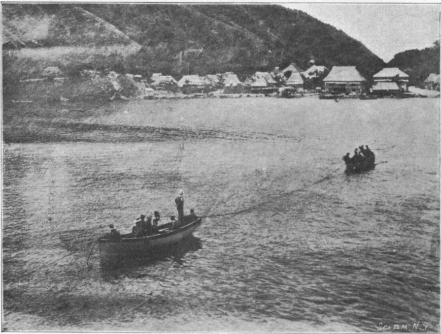
Landing the End of a Cable by Small Boats.
