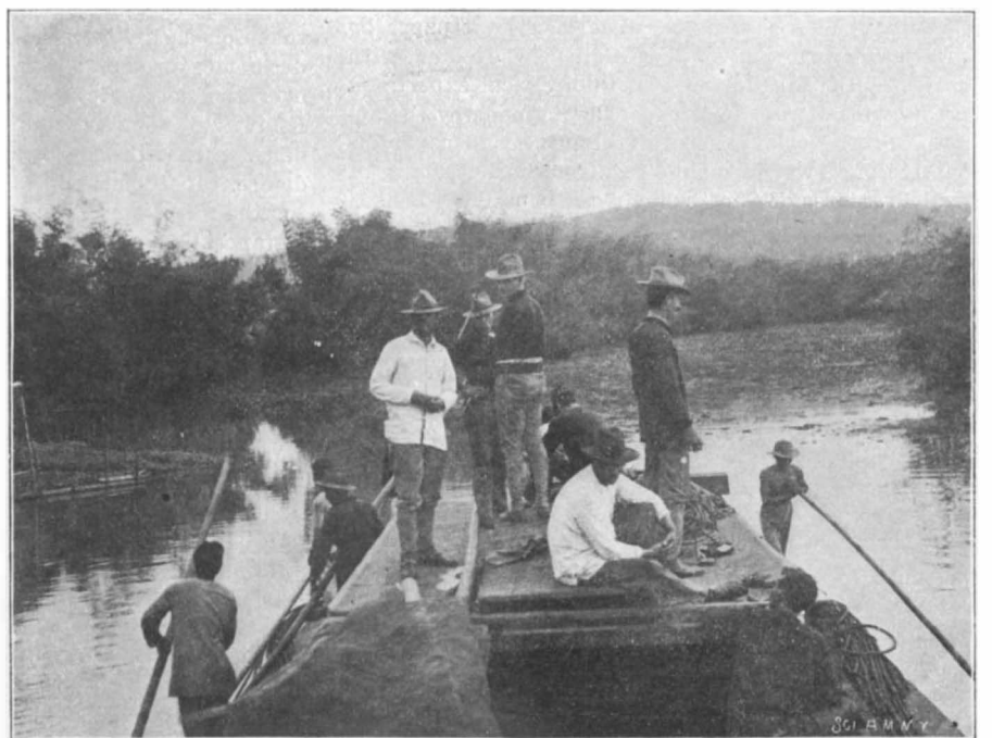
Laying Cable from Barge Up a Small River.
