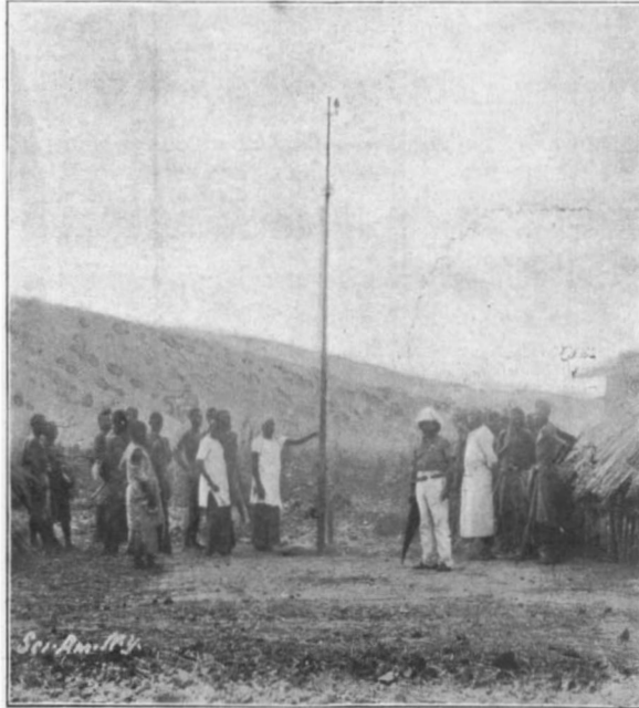
ERECTING THE FIRST POLE IN GERMAN EAST AFRICA ON THE RHODESIAN FRONTIER, SEPTEMBER, 1900.
