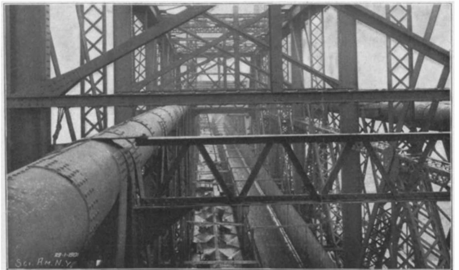
Old and New Trusses During Construction.
