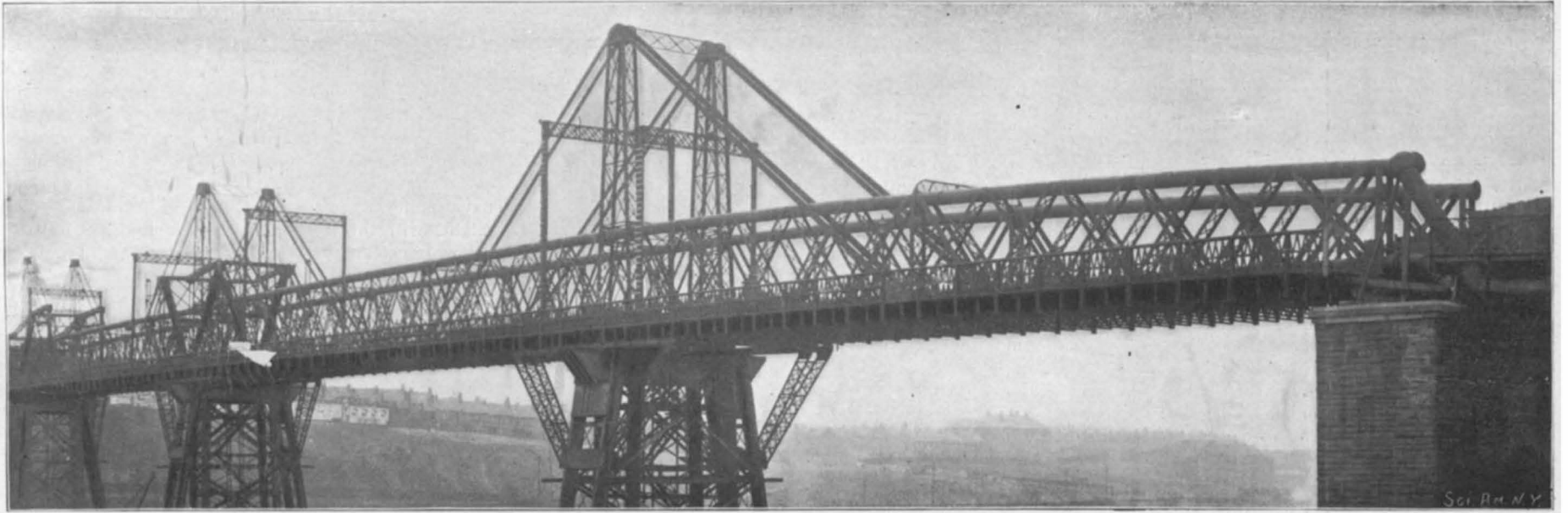
The Old Bridge—Top Chords Utilized as Gas Mains, Bottom Chords as Water Mains.
