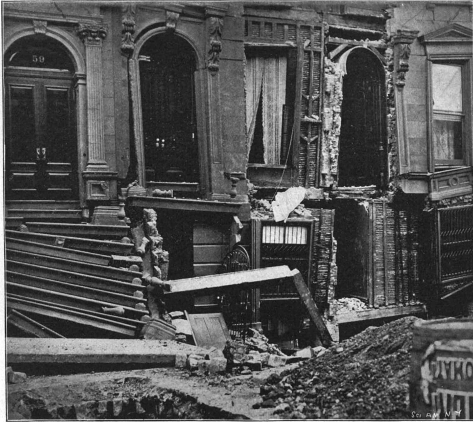
Front View of the Wrecked Houses.
