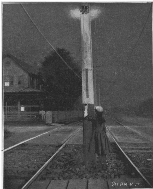
Fig. 1.—SETTING THE NIGHT SIGNAL FOR A TROLLEY CAR.
