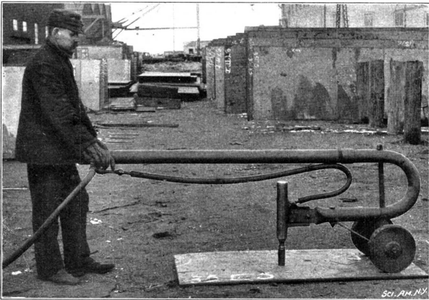
DECK RIVETER IN POSITION.
