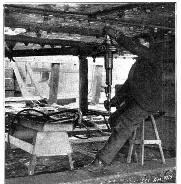
SHELL RIVETER WORKING ON THE BOTTOM.
