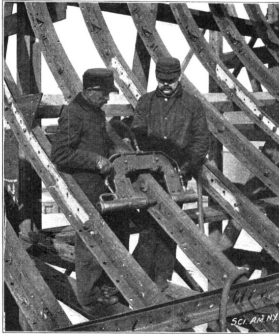
RIVETER AT WORK ON SIDE FRAMING.
