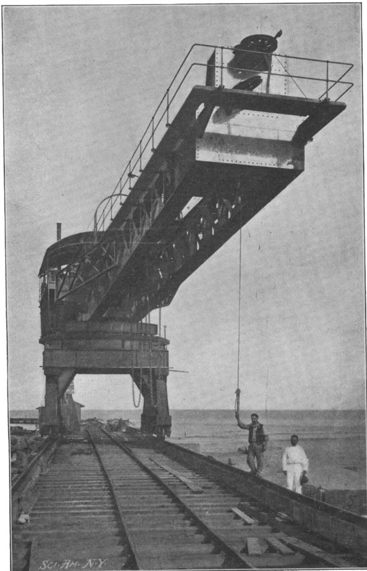
The West Breakwater Crane.
