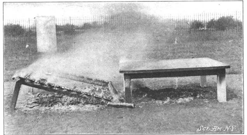
AFTER THE FIRE. WOOD PLATFORM DESTROYED, URALITE PLATFORM INTACT.
