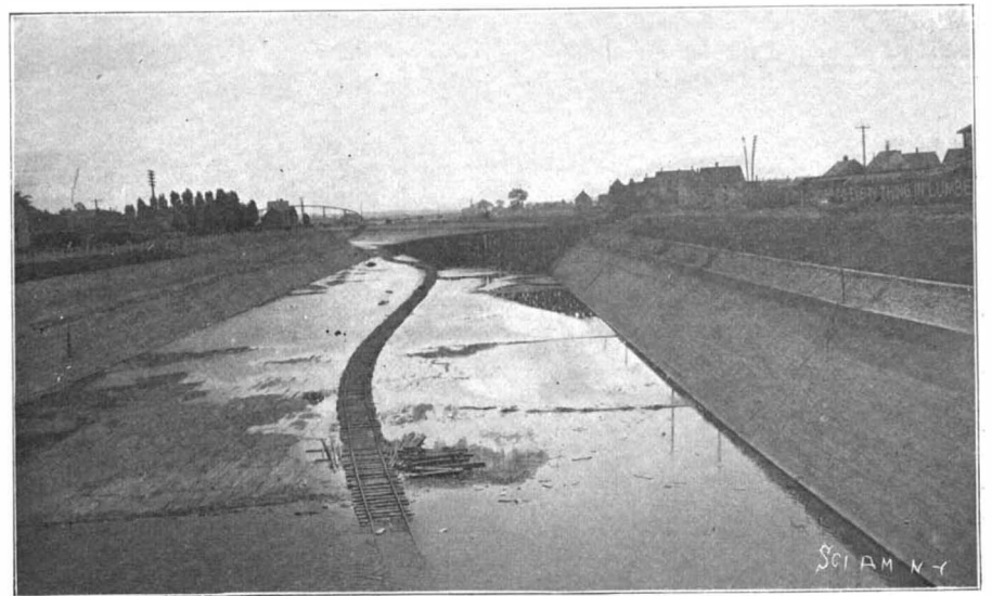
A Stretch of the Canal, Showing Highway Bridge in the Distance.
