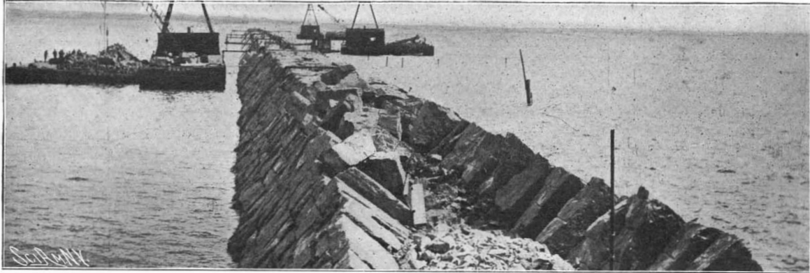
Finishing Off Stone Breakwater with Heavy Top Angle Stones.
