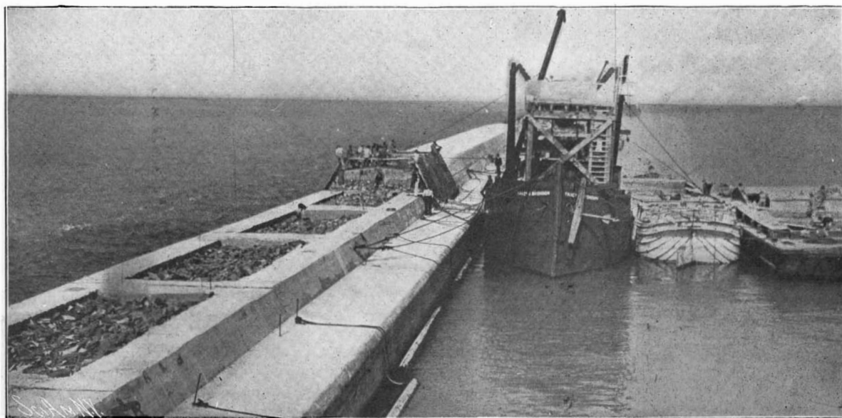
Building Concrete Structure Above the Timber-crib Foundation.
