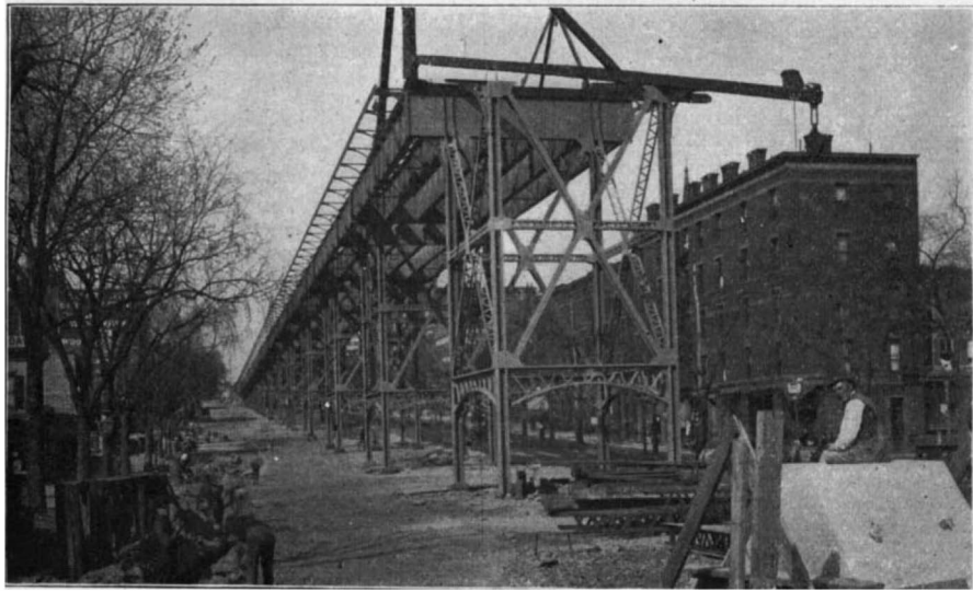
Manhattan Valley Viaduct, Showing Skewbacks for Arch.
