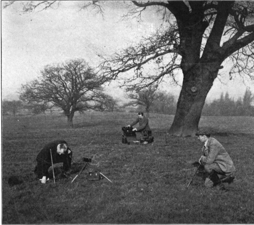
ORE PROSPECTING BY MEANS OF ELECTRICITY.
