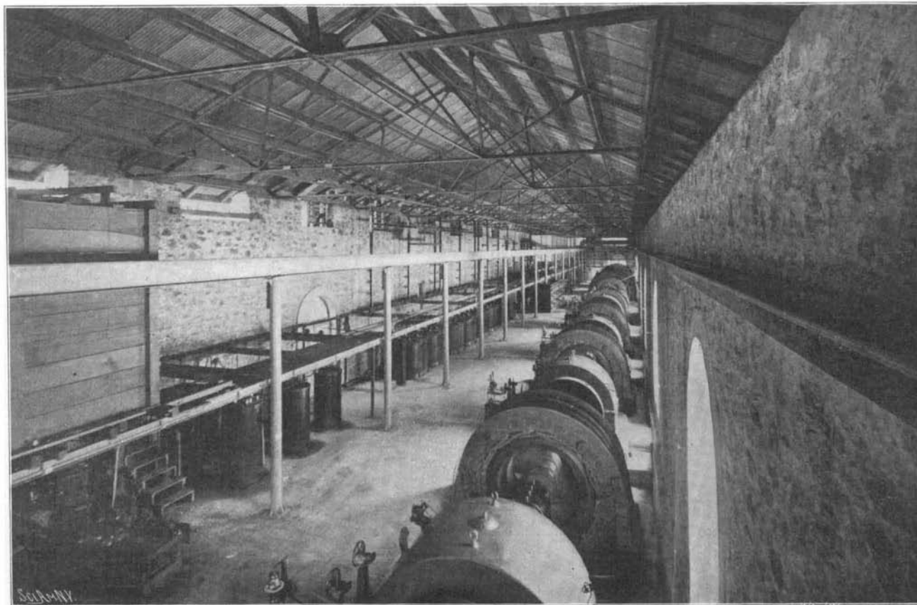
The Latest View of the Interior of the Colgate Power House.
