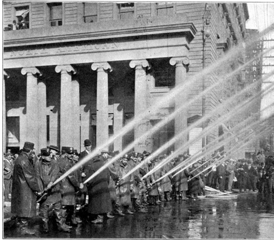
Twelve 2-Inch Streams of Water, Thrown 200 Feet.
