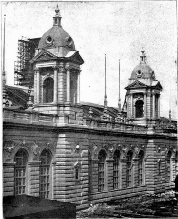
Finished Portion of Machinery Palace.
