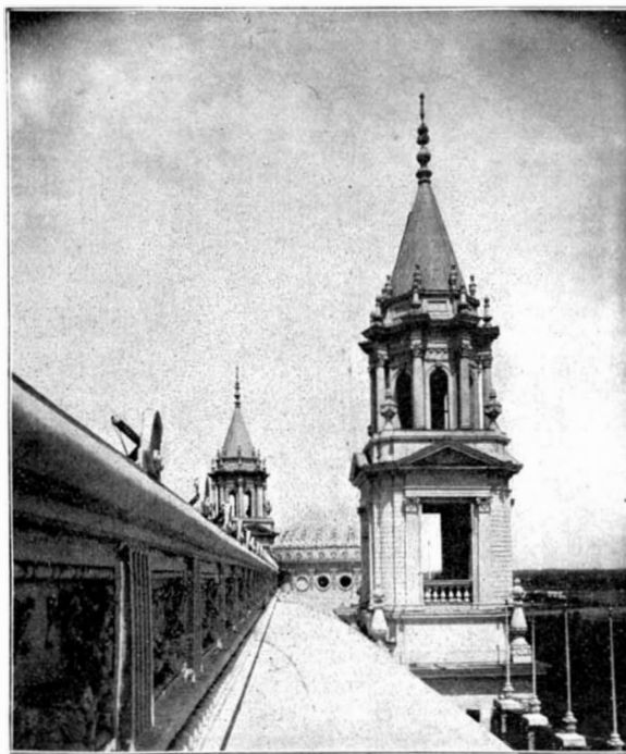
One of the Towers of the Palace of Varied Industries.
