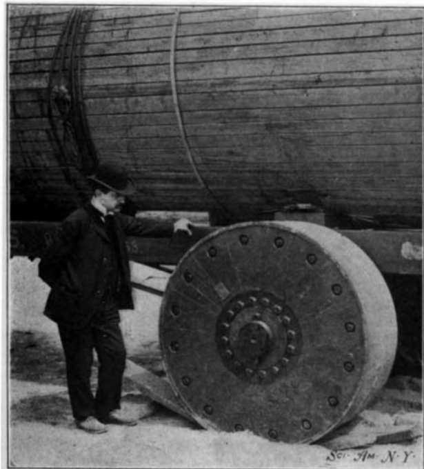
Rear Wheel Embedding Itself in the Ground.
