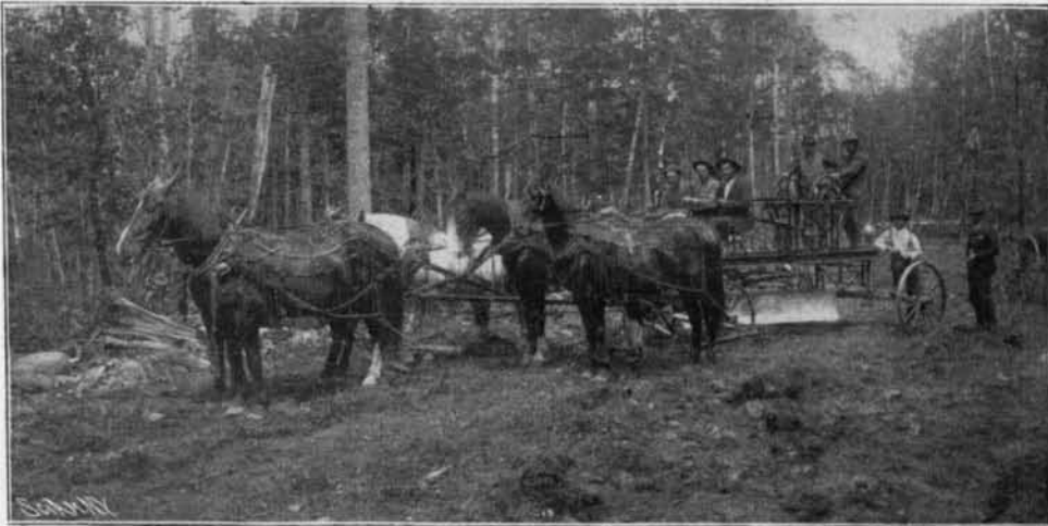
Road-Making at Hayward, Wis.
