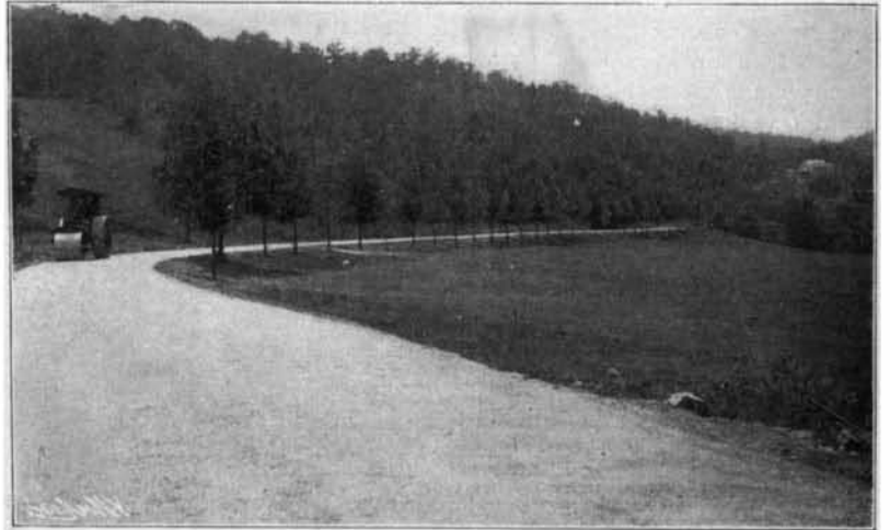
A Finished Road at Hot Springs, Va.
