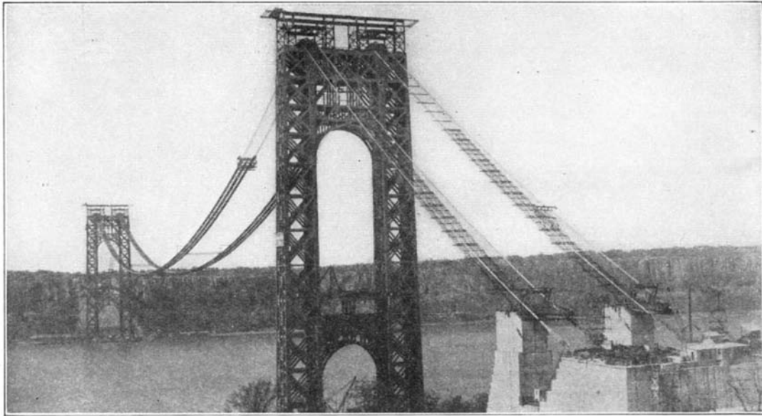
ALMOST READY FOR SPINNING THE CABLES
