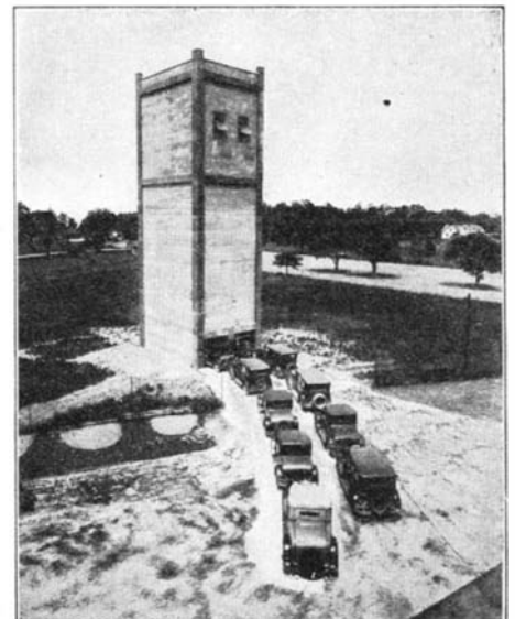
Car parking tower, an independent invention which is operated on practically the same principle as the one described and illustrated above. It was invented by Mr. J. E. Morton of Sandusky, Ohio
