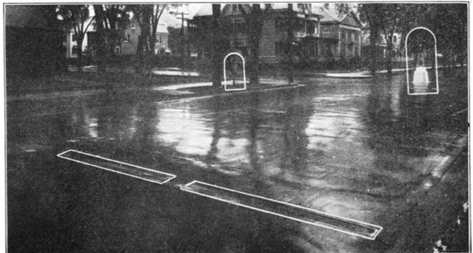
Automobiles passing over the pavement installation outlined in foreground "notify" the control, in center background, which operates lights at right
