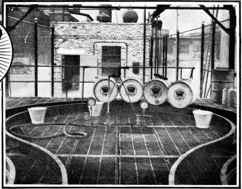
Below—Close-up of Ethyl mixing plant. Drums on runway contain Ethyl fluid about to be mixed with gasoline to form Ethyl Gasoline.
