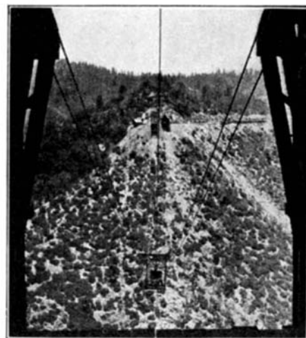
View from receiving and control building showing aerial tramway cable carrying a heavily laden car
