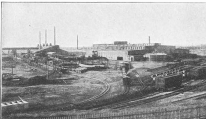
ELECTROLYTIC COPPER REFINING PLANT
