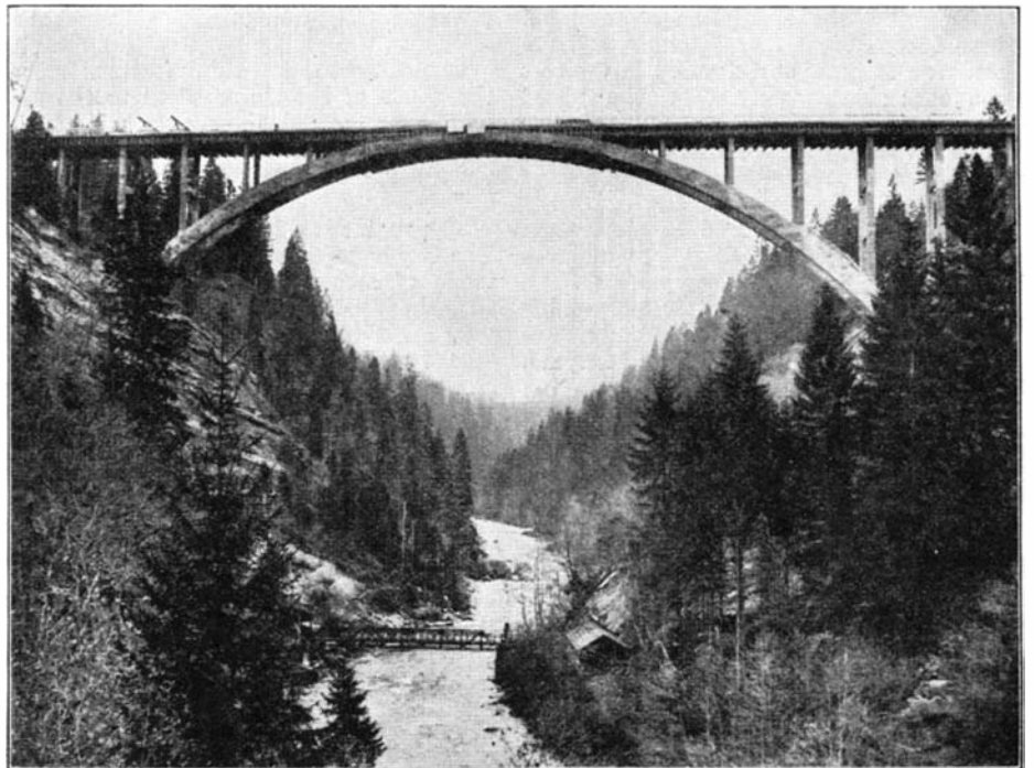
Near Echelbach in South Bavaria, this bridge, which is nearly complete, is said to be the highest concrete bridge in the world. It is 597 feet long, 246 feet high, and has a width of 52.5 feet. Built especially for automobiles, it will expedite vehicular traffic to the Passion Play at Oberammergau in 1930
