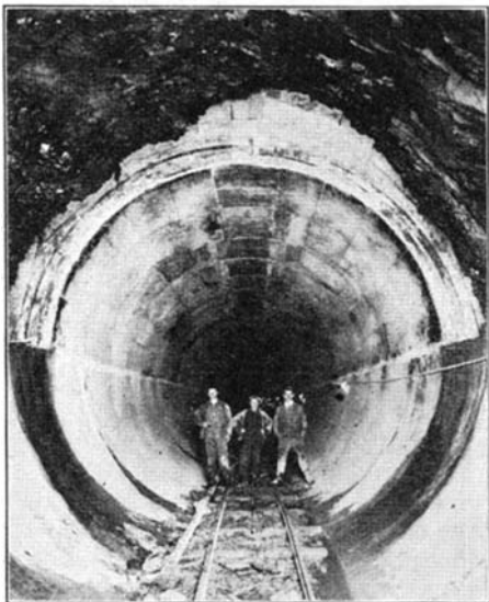
A tunnel of the New York City water supply system. The tunnel being built will be even larger
