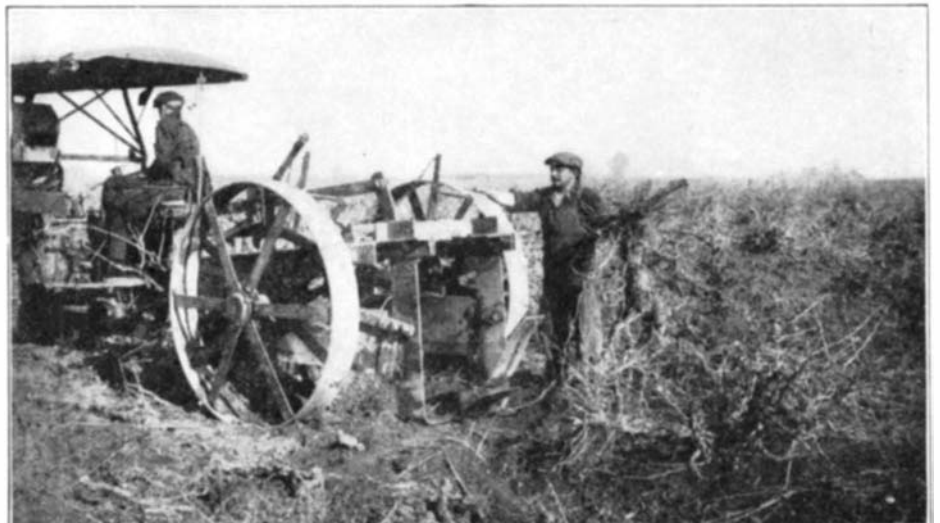
The sub-soiler equipment is useful also for uprooting the matted and gnarled roots of old worn-out vines when necessary to replace them with new ones
