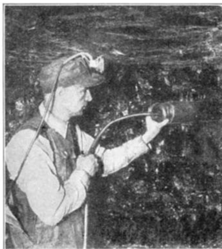
INSERTING CABLE TERMINAL
