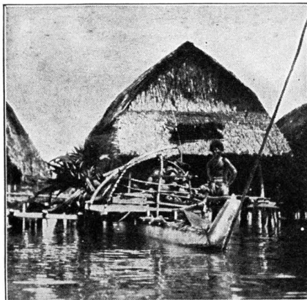
BUILT ON PILES
