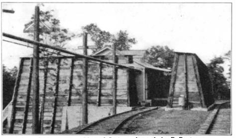
Gelatin cartridge house, Mineral Springs plant of the DuPont company, showing earth barricades which serve as protection in case of explosions
