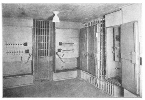
Control compartment enables a guard to direct the movements of 39 detained persons. Doors to cells are opened and closed mechanically from this station
