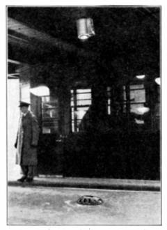
The photoelectric cell in the roadbed and the light source overhead
