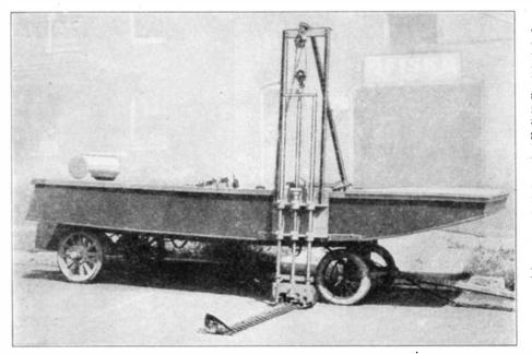
The lily mower which cuts the stems of these plants under water. It consists of a boat (here shown on wheels) with an adjustable mower attachment
