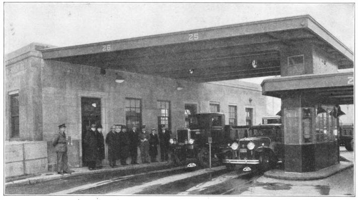
A toll house showing photoelectric cells in roadbed and lights overhead
