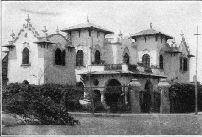
First glance at this Moorish type adobe house in Lima, Peru, would give the impression that it is of plaster
