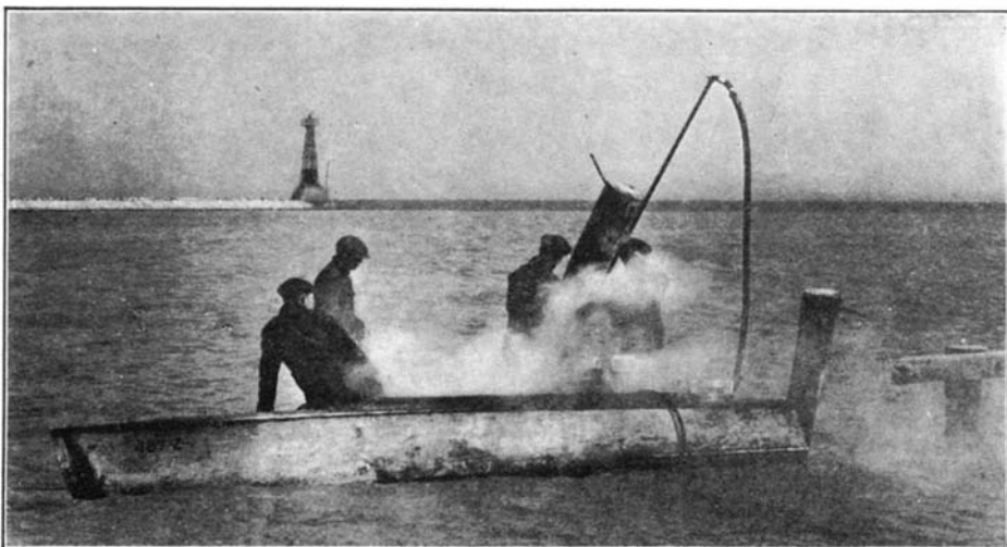
Removing piling with outboard-powered high-pressure pump
