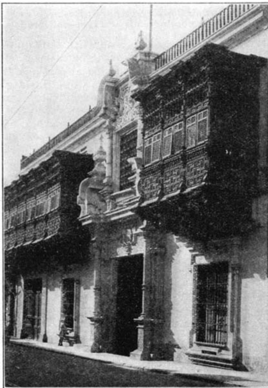
A mud building that has stood for over three centuries. The Torre Tagle Palace
