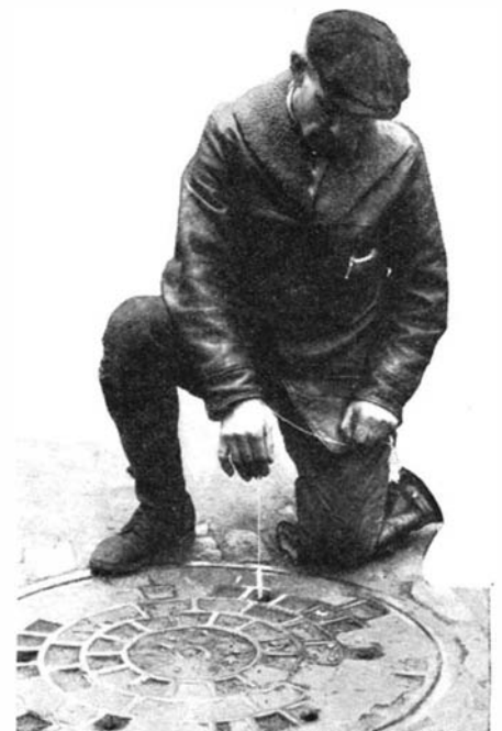
Testing for carbon monoxide gas in a manhole with an ampoule
