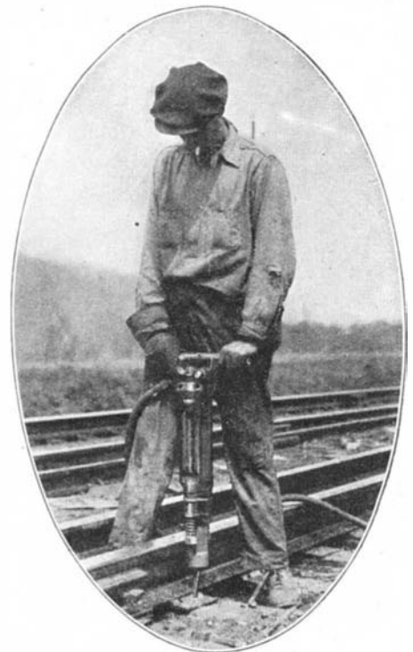
A pneumatic hammer speeds the work of driving spikes into the ties
