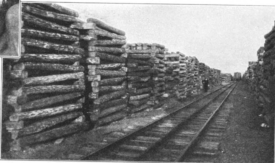
Railroad ties by the thousands are stored in piles ready for use in the laying of new track or replacing old ties. Most of the ties are chemically treated
