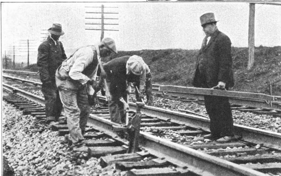
Here the hand tampers are elevating the track slightly where necessary. This leveling prolongs the life of track. The track gage is always in use
