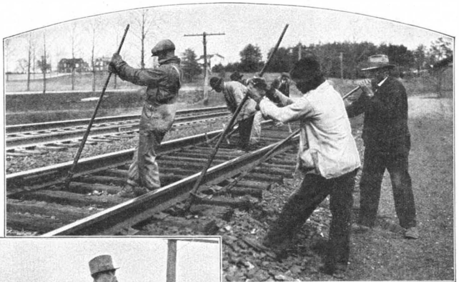
Rails are elevated to proper position by hand jacks. The tampers then follow, tamping the ballast under the ties to make a firm foundation
