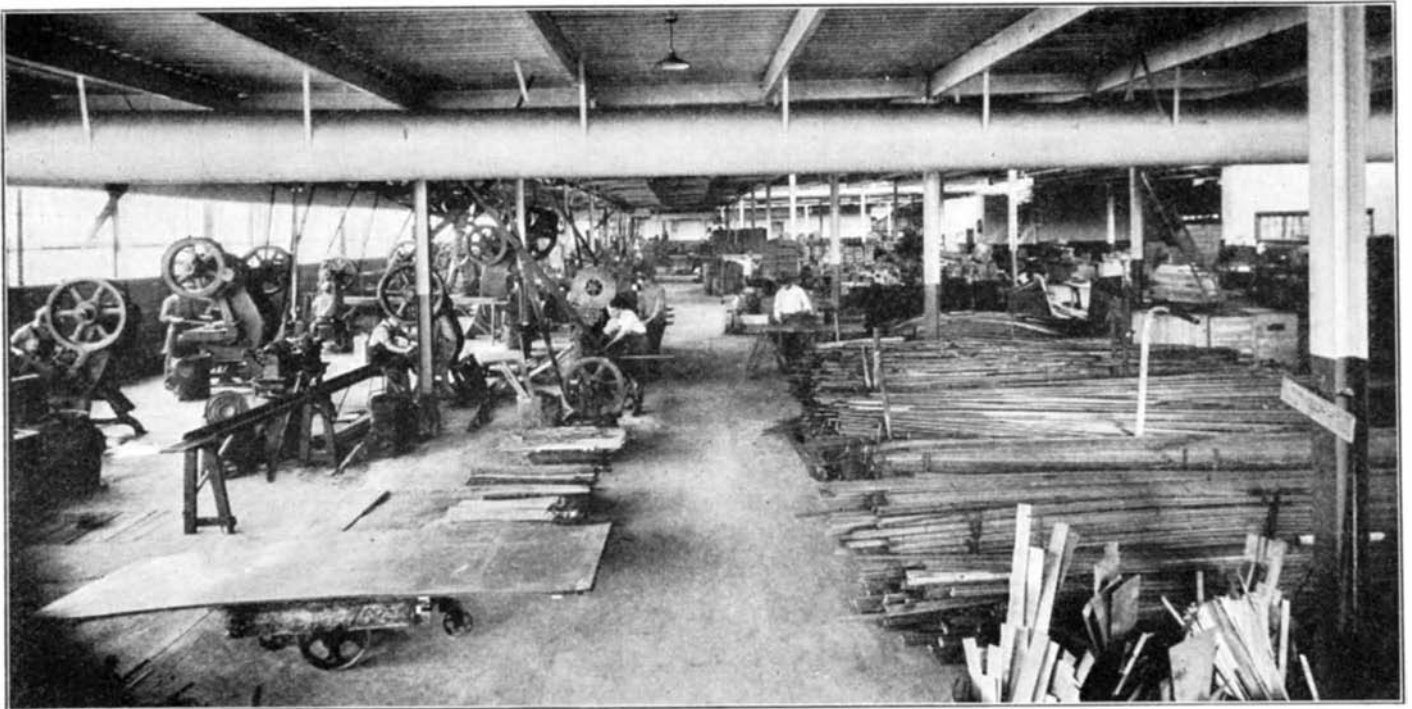
Nothing but toys are made here. Interior view of a large plant which manufactures toy aircraft. Large supplies of raw materials are in the foreground, and the lines of presses for stamping out parts are visible at the left
