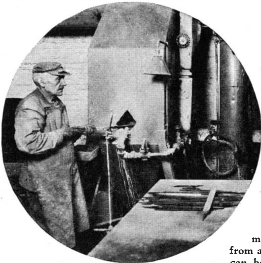
Reclaiming used files by the steam sand-blast method. Approximately 15,000 files a month are reclaimed at the East Pittsburgh plant alone
