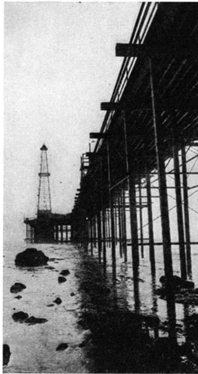
Far out beyond low tide level— one of the completed oil derricks
