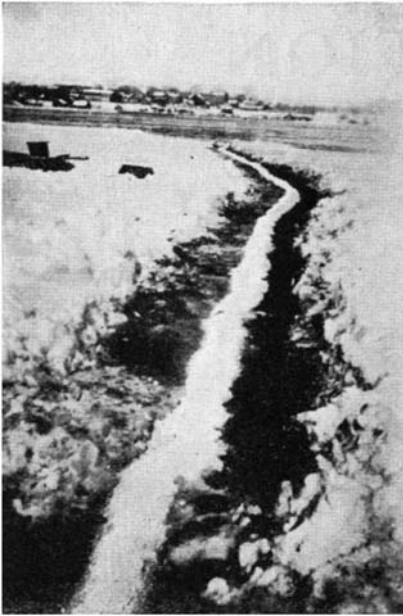
Ice in the ship channel of a river "rotted" away and a clear channel being made with calcium chloride
