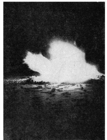
Destroying an ice jam with 12 pounds of solite, the new chemical which is "touched off" by water
