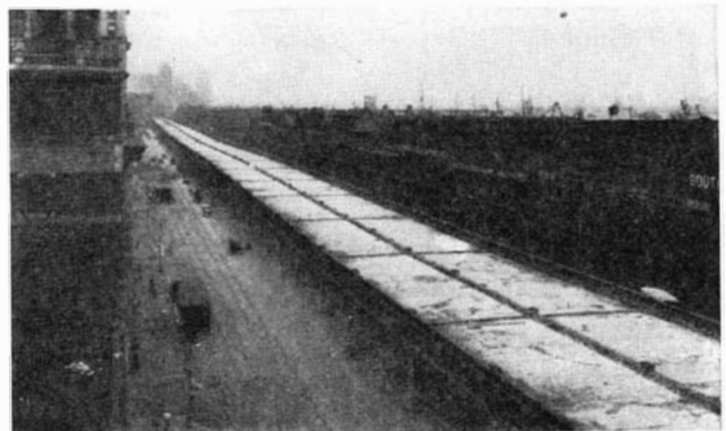
Nearing completion: lower section with paved roadway
