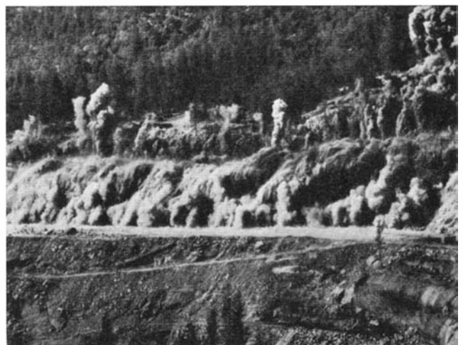
The same cliff "erupting." When this blast was made, stone totalling 231,700 cubic yards crumpled from its face
