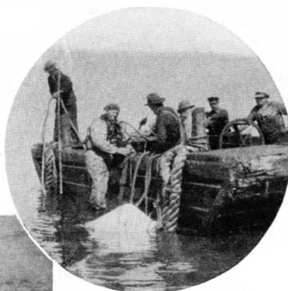
To facilitate its progress over the ocean floor, the forward end of the pipe-line was equipped with a sled. The pulling bridle is here shown in place
