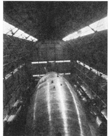
The metal-clad airship in the hangar where it was built. Its metal "ribbon" construction is shown
