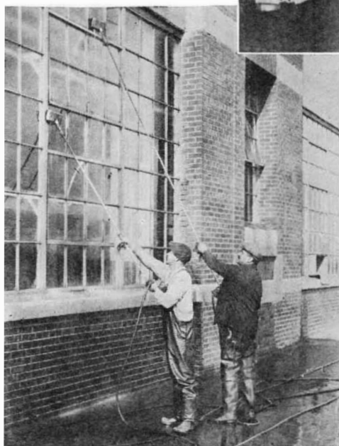
Windows are kept clean. The brushes have hollow handles to convey the water
