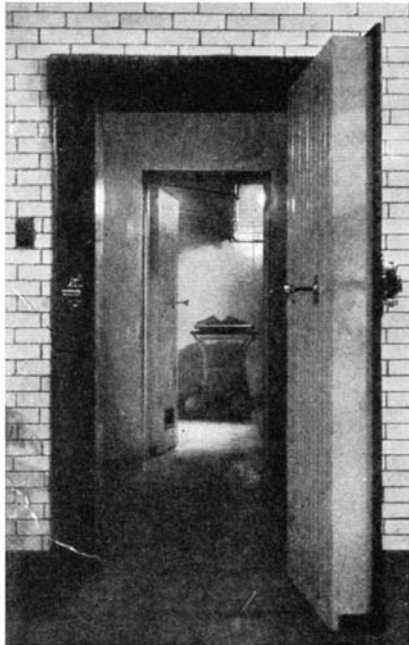
The "zero room" is separated from the crypts by an isolating air lock
