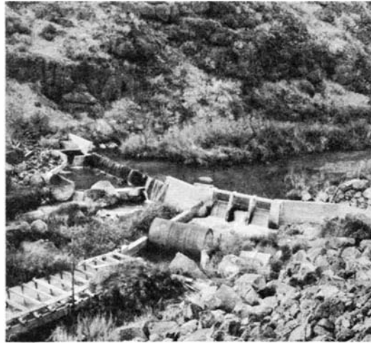
Courtesy California Fish and Game Commission Rotary fish screen on an irrigation ditch and, at far end of dam, a three-jump fish ladder
