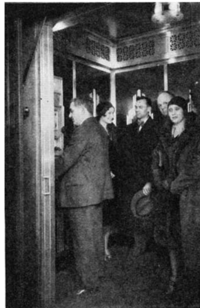
View of car and control board. Car is made of aluminum and Micarta, reducing weight and running costs. See the text below
