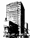
State-Planters Bank Building, Richmond, Virginia.—"Iron Fireman has cut our fuel bill in half. There is also saving in labor as the machine is fully automatic, affording more uniform heat and constant boiler pressure."
