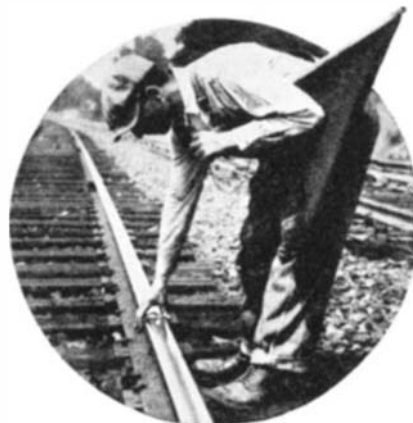
A torpedo is clamped to the rail and is detonated by the locomotive
