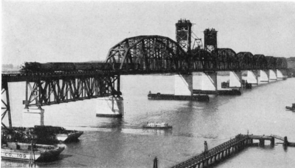
Southern Pacific's 5603-foot double-track bridge across Suisun Bay in California. Costing a total of 12,000,000 dollars, it was completed in the fast time of eighteen months
