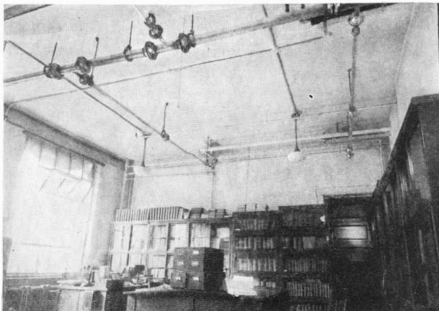
Pyrex pipes running through the office of a chemical plant enable an executive to keep a constant check on the color and so on of liquid flowing through them
