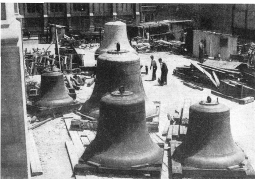
The new bells for the Riverside Church. The "bourdon" weighs 20½ tons and is swung and struck at different times. The larger bells are placed below the console
