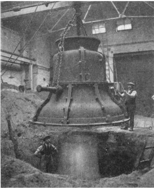
Lowering the case onto the core in the pit before casting
