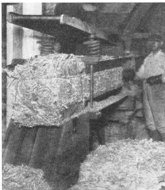
A specially designed extra heavy baler turns out a 250 pound bale of bagasse
