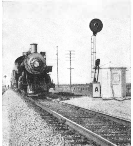
When necessary to communicate with the dispatcher, the telephone in the little house is used
