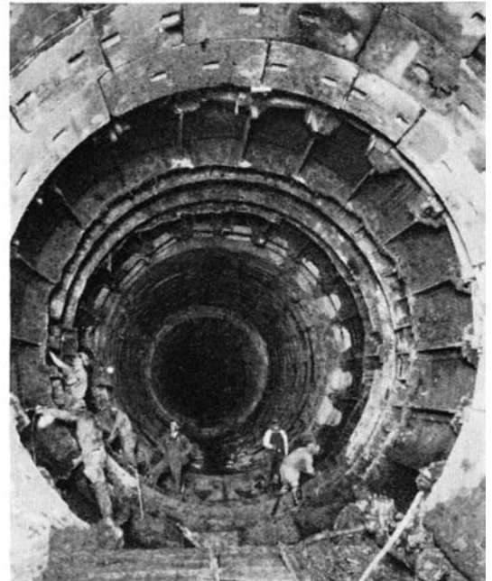
At left: Front view of one of the hydraulic block erectors, showing the manner in which the huge blocks weighing over a ton each were placed in position
