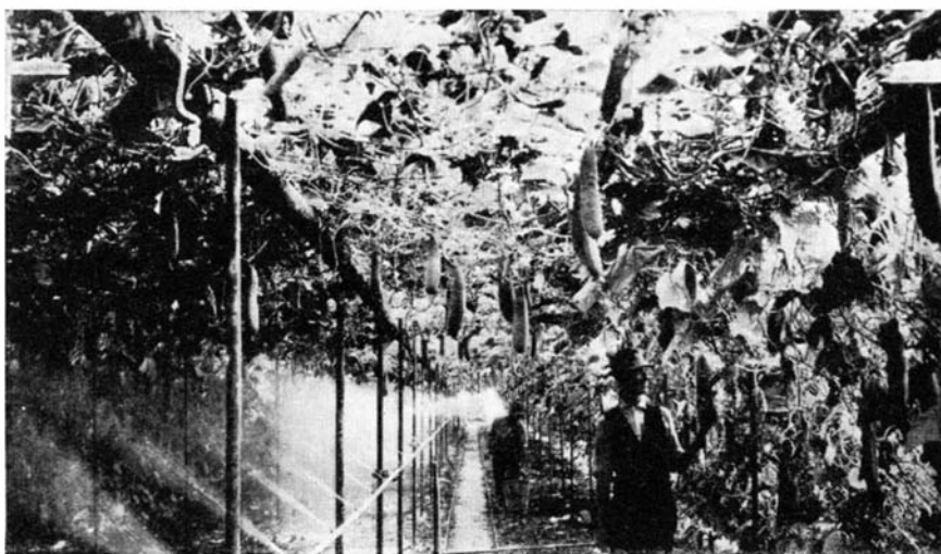
A profitable crop of choice greenhouse cucumbers showing the stick and overhead wire-mesh support. Notice the sprinkler irrigation pipe in operation
