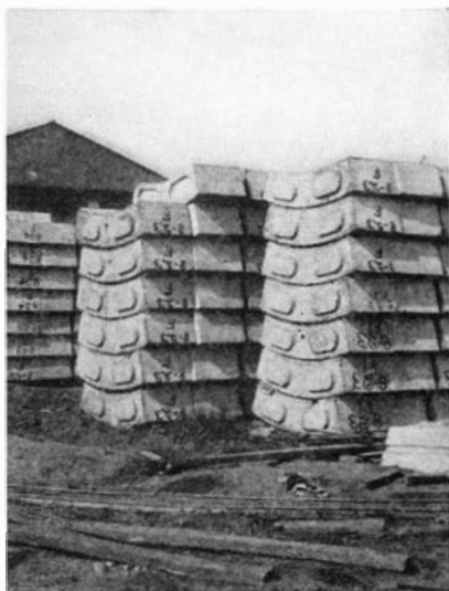
A total of 45,790 of these ring blocks was used in the new tunnel
