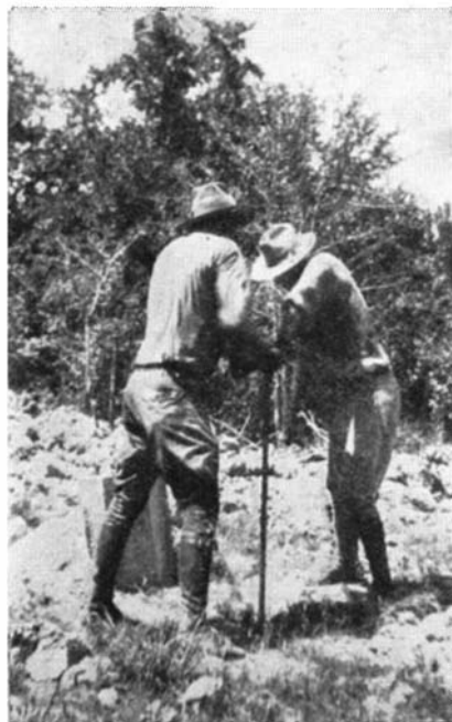
The dynamite crew making a 20-foot hole into which, after enlargement, 300 pounds of dynamite will be put
