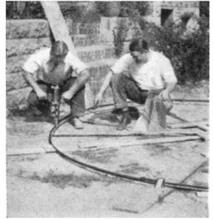
Figure 4: The fixed track of angle iron, after being bent, was drilled
