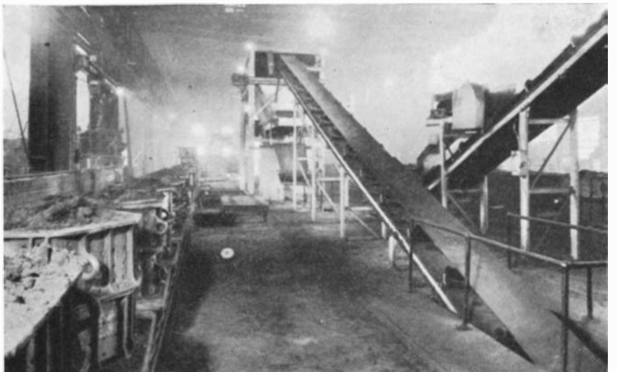
The belt in foreground elevates sand to sandarator and hopper over sandslinger. The one in background carries sand from shakeout and separator to sand muller
