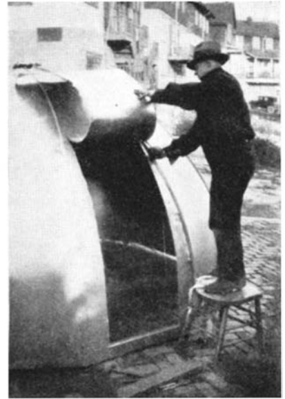
Figure 9: Cutting out the opening for the shutter was the next thing
