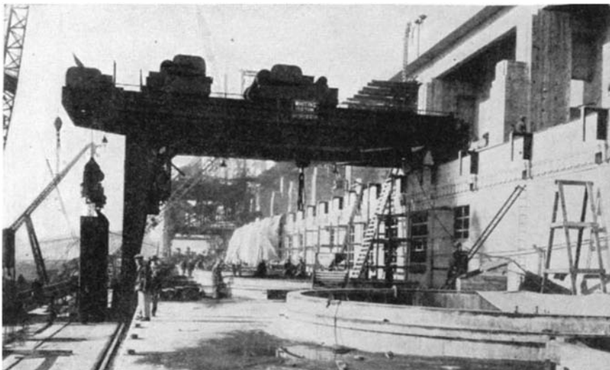
A gantry crane capable of lifting 150 tons can be placed over any generator to assist in repairs or, if necessary, to remove both generator and water wheel
