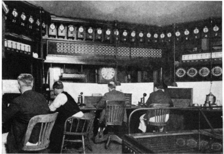
The operators in the dispatcher's office at Tower K, Washington terminal, give orders to the levermen who operate the switches and signals, all interlocked
