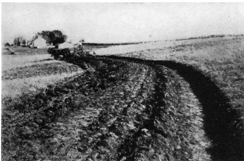
A terrace nearly completed in North Carolina. Following the contours of a field, terraces such as this prevent the downhill rush of soil-washing rainwater
