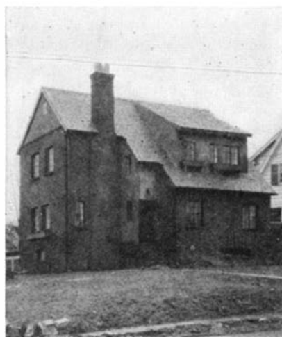
The completed dwelling with frame made up of welded steel panels
