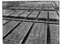
The St. Louis University's School of Commerce & Finance. Gillespie & Daley, contractors, used 60,000 sq. ft. \frac{1}{4} " Presdwood as concrete forms for 150,000 sq. ft. area, producing smooth surface concrete of notable strength. The 3' x 12' pans permitted saving in concrete due to their size
