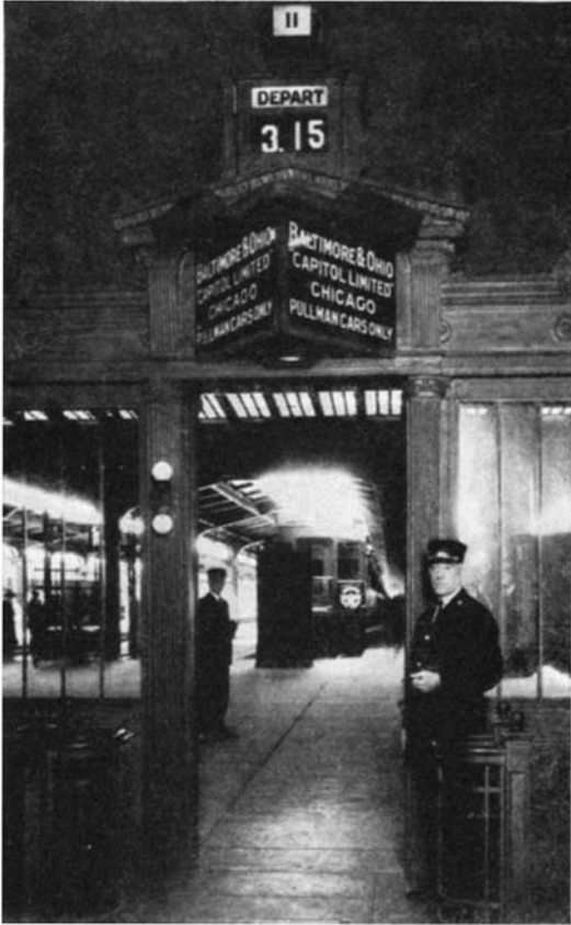
Gate showing the twin lights at the left which play an important part in all train departures
