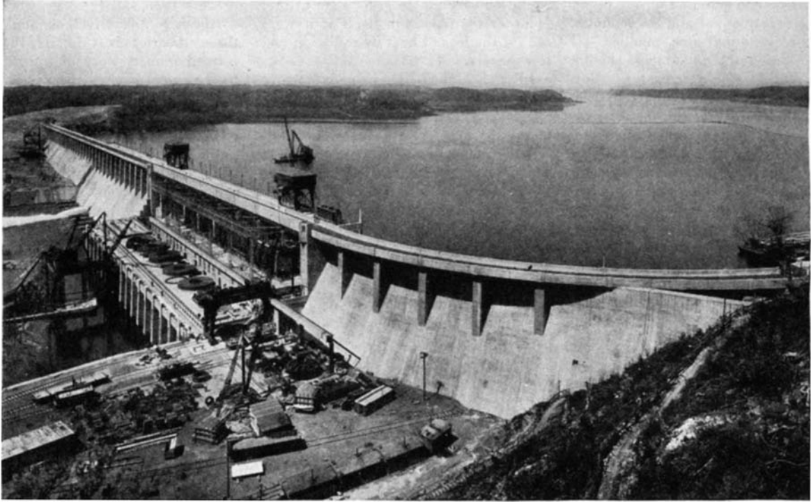
The Bagnell Dam not only impounds 87 billion cubic feet of water—sufficient to generate about 425 million kilowatt-hours of electricity annually—but also serves as a bridge over the Osage River
