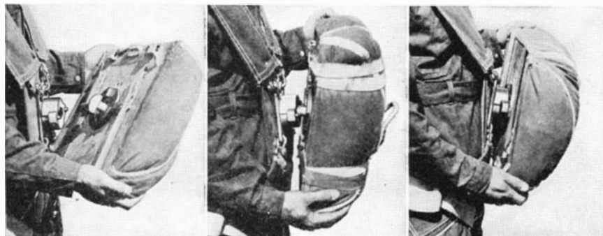
Using the quick-attachable parachute holding device. The airman is ready to jump after placing the fittings together and giving the pack a quarter turn
