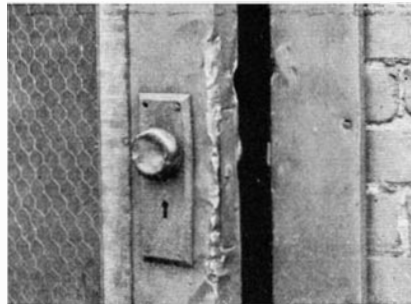
Left: The right way to open a door is to get an honest locksmith to pick the lock. It requires great skill and experience and special tools and no amateur need apply. Upper: The trail of the "jimmy." Right: The wrong way to open a door—jimmying a loft door is also very hard work
