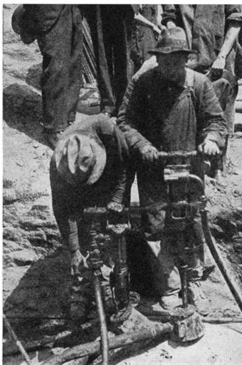
Dust cap at the base of each drill is attached to an air suction system by a hose
