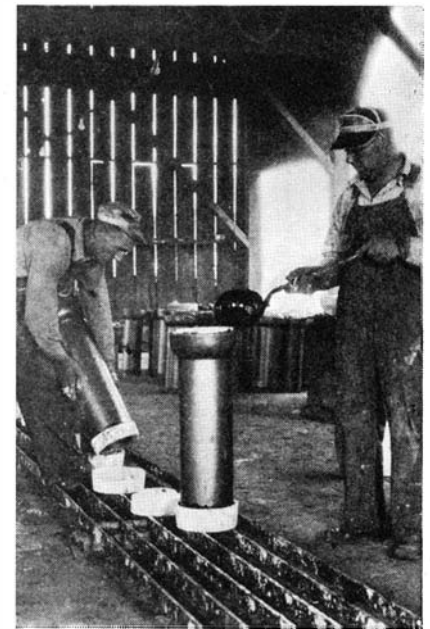
Hot asphalt being poured in making efficient pre-cast sewer pipe joints
