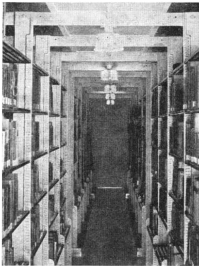
Specially designed perforated light shades protect stack attendants from glare yet illuminate shelves
