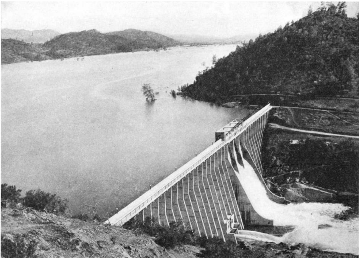
The Stony Gorge Dam which stores up a wealth of water for the Orland Project, California, and thus has all the potentialities for the production of luxuriant crops and the consequent prosperity of farmers
