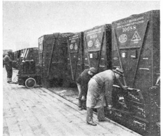
The process of lowering the sectional sides of the car is simple. Each forms a gangway
