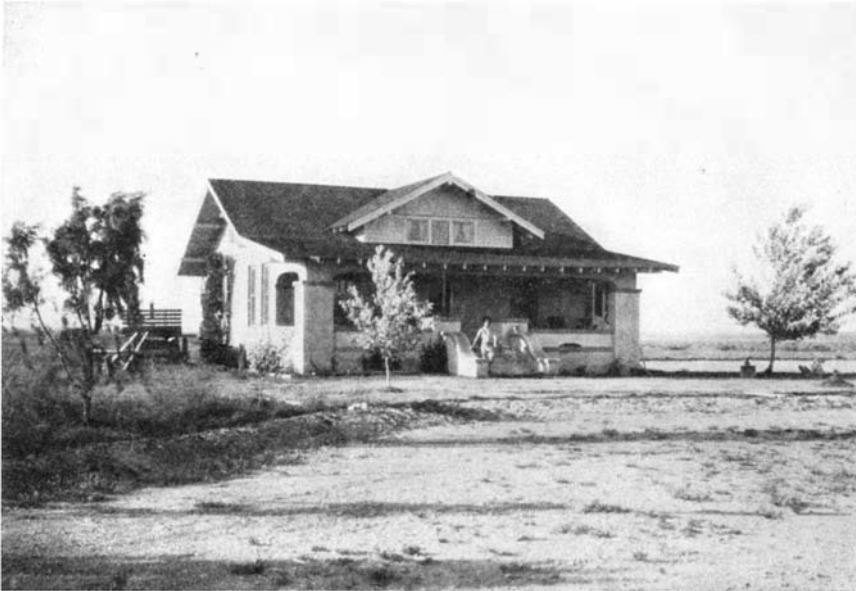
The glistening silver that is not mined but flows in ditches made possible this up-to-date home of an irrigator-farmer on the Carlsbad Project, New Mexico
