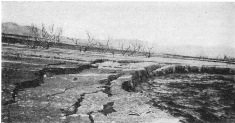
The waters of the Salt River cutting out silt in the upper part of the Roosevelt Reservoir basin, and carrying it nearer to the dam
