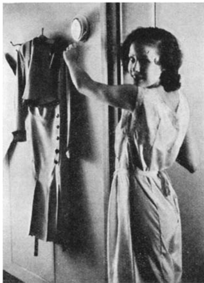
The new wall light, operated by a pull chain, in use in a closet
