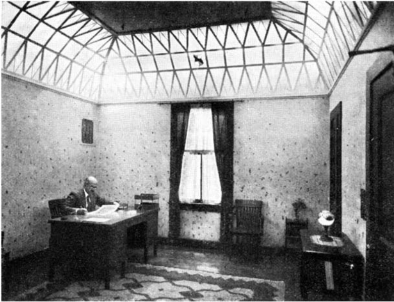
Left: The windowless office is a coming reality. We will work in an air-conditioned room flooded with artificial light from unobtrusive sources. In the center of the ceiling is an ultra-violet unit, while the window is false, being lighted by a blue daylight lamp. Right: Auxiliary illumination projected from built-in system with a daylight lamp back of a prismatic glass plate
