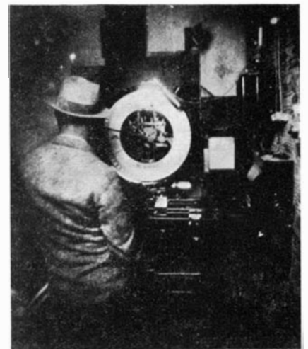
The operator who checks the materials for the concrete of Koon Dam
