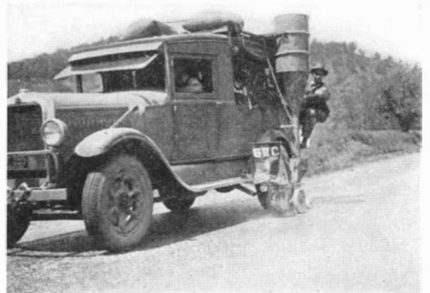
The manner in which the paint spray gun and the tank of blotting sawdust were mounted on the car
