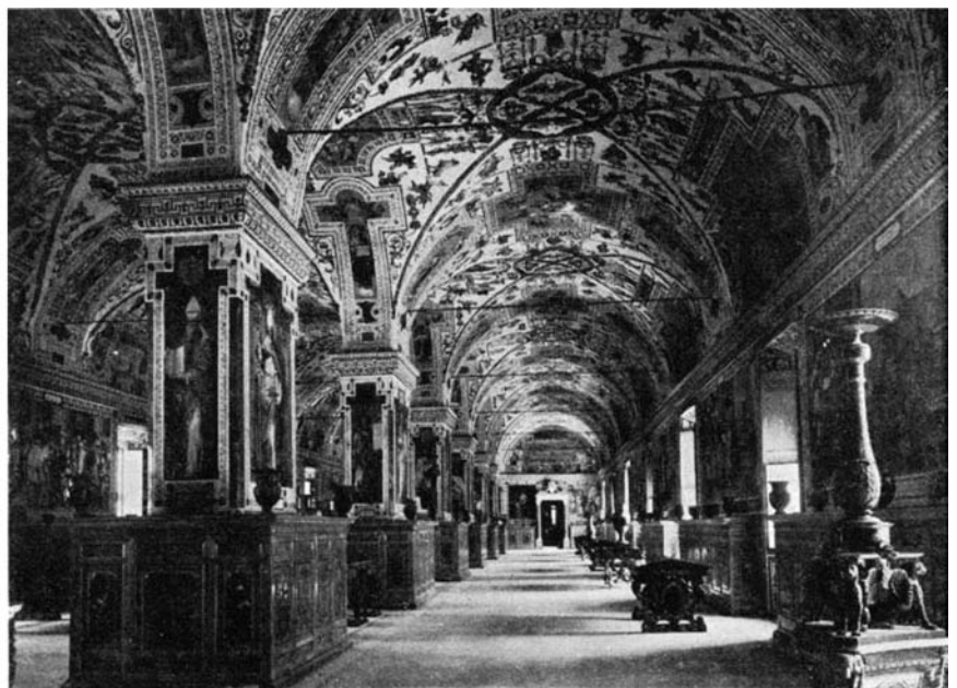
The superb Sala Sistina, a section of which was destroyed by the collapse of the roof, destroying 1000 rare books, damaging many more, and killing five persons
