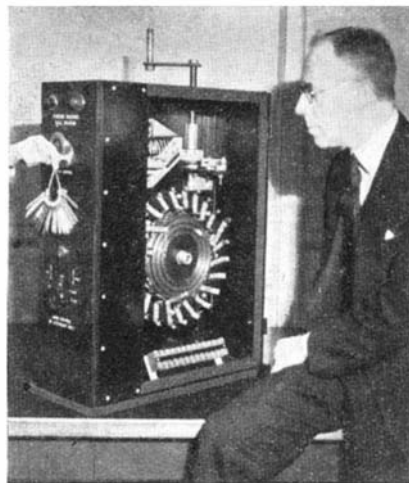
Twenty-four keys make this lock perform 24 different operations
