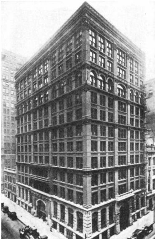
A world-famed architectural milestone: the old Home Insurance Building, Chicago
